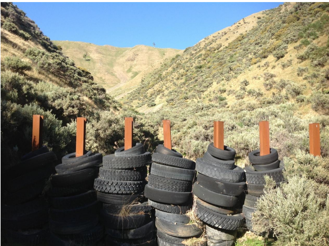
Photo 18: Debris collector at the bottom of Hill Road Gully
